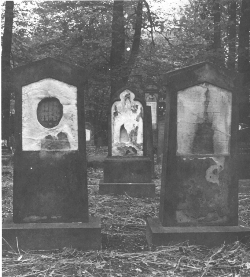
Fig. 2. The damage caused to grave monuments at the Mosaic Cemetery in Copenhagen.
