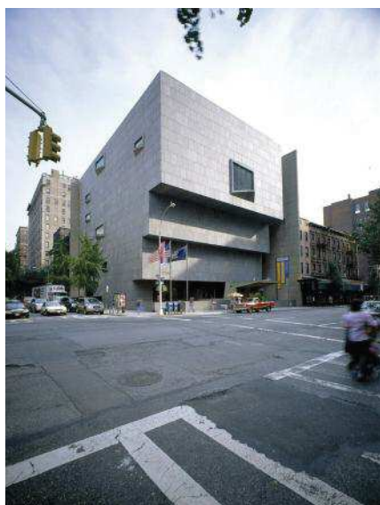
Fig. 7 Whitney Museum, Upper East Side, 75th Street and Madison Avenue, Photograph by Jerry L. Thompson.
