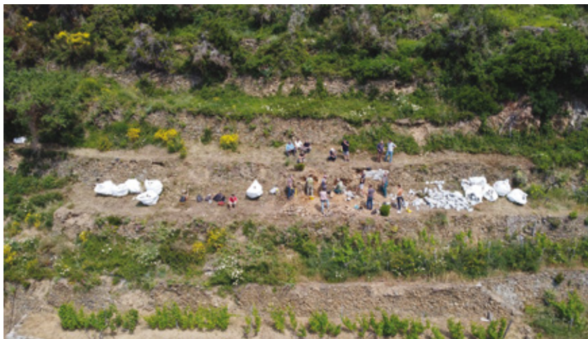
Dry-stone wall reconstruction and restoration in the Cinque Terre National Park © Parco Nazionale delle Cinque Terre (Emanuele Raso)
