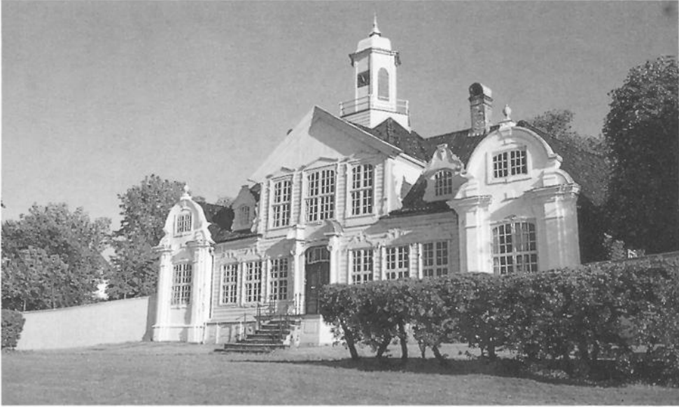
Fig. 1. The Rococco building of Damsgård from about 1780 seen from the north. The miniature Baroque garden lies close to the main house on the left, and a carp-pond and a duck-pond to the right (Photo T. Indahl).
