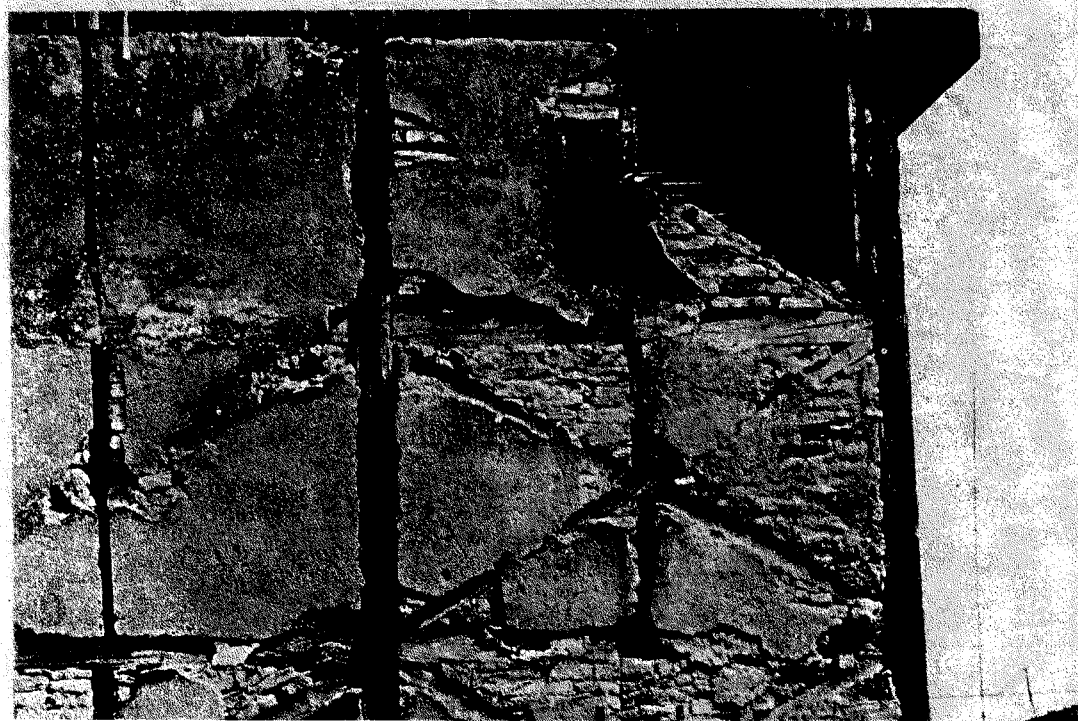
Plate 3 Damaged walls of "case baraccate" in Reggio Calabria. (from: C. Barucci, op. cit. )
